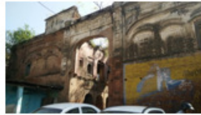
Fig. 6. Purani Haveli- a old dilapidated structure in Mansar lake.
